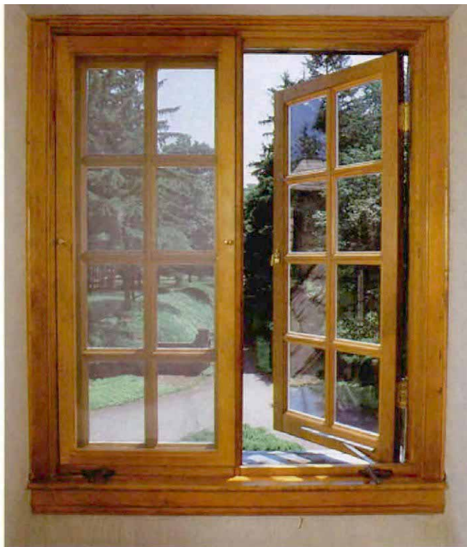
The slotted track and crank housing of the casement operator are simply screwed in place. The "crank molding" is the narrow stock notched to fit over the crank housing. It provides a surface for the screen to sit on. The solid-brass hinges have a small set screw in the barrel that prevents the hinge pins from being removed from the outside.
